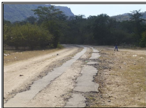
Strip road remnant - Zimbabwe 2015 (Photo “Mike”)
